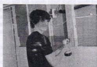
Graham Houghton, Carpenter/Renovator for Stagecoach Properties
