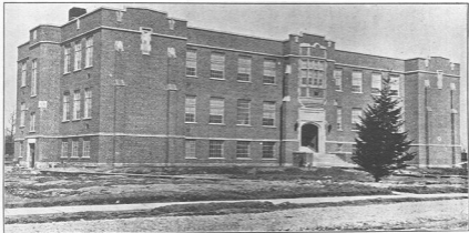
PORT CREDIT HIGH SCHOOL, 1930
